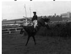
Foinavon – Fence 7 and 23 Height: 4 feet 6 inches {1.37m}
